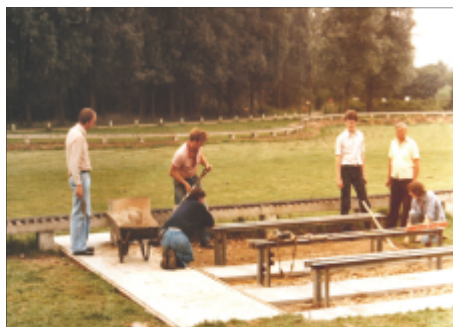
Steaming bays were constructed.....
